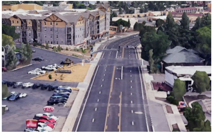
LOOKING EAST AT THE INTERSECTION OF PINNACLE ST.
